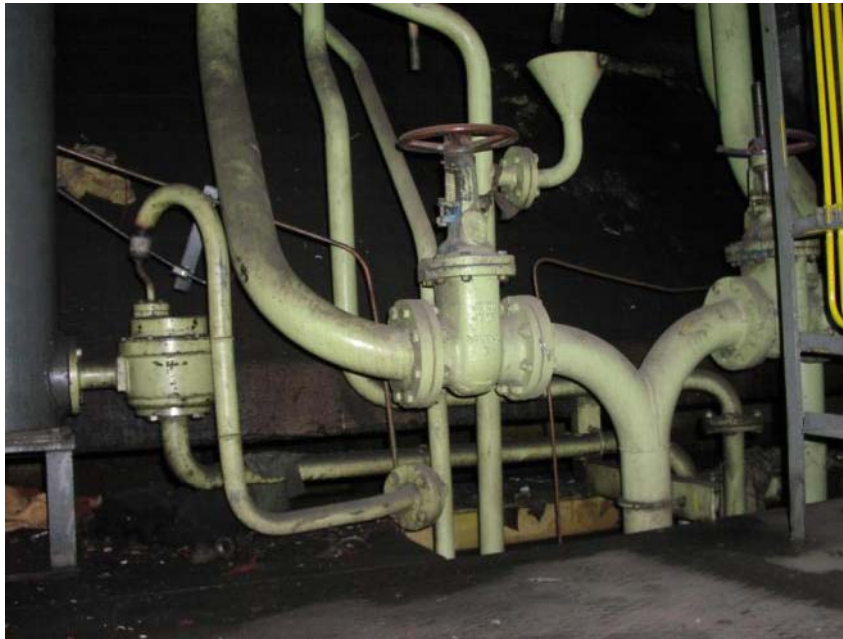
Water system before
